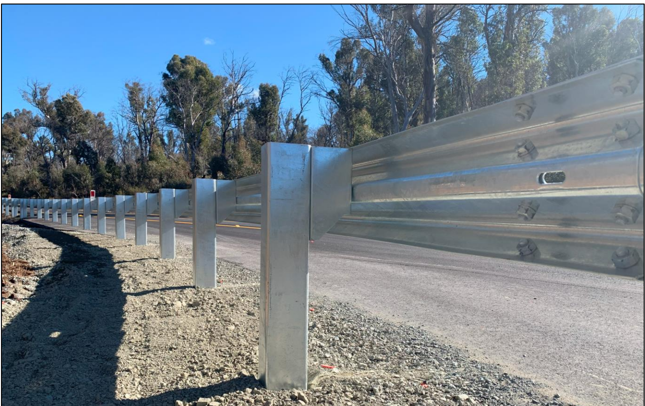
Figure 16: Horizontal Curving of W-Beam Guardrails
