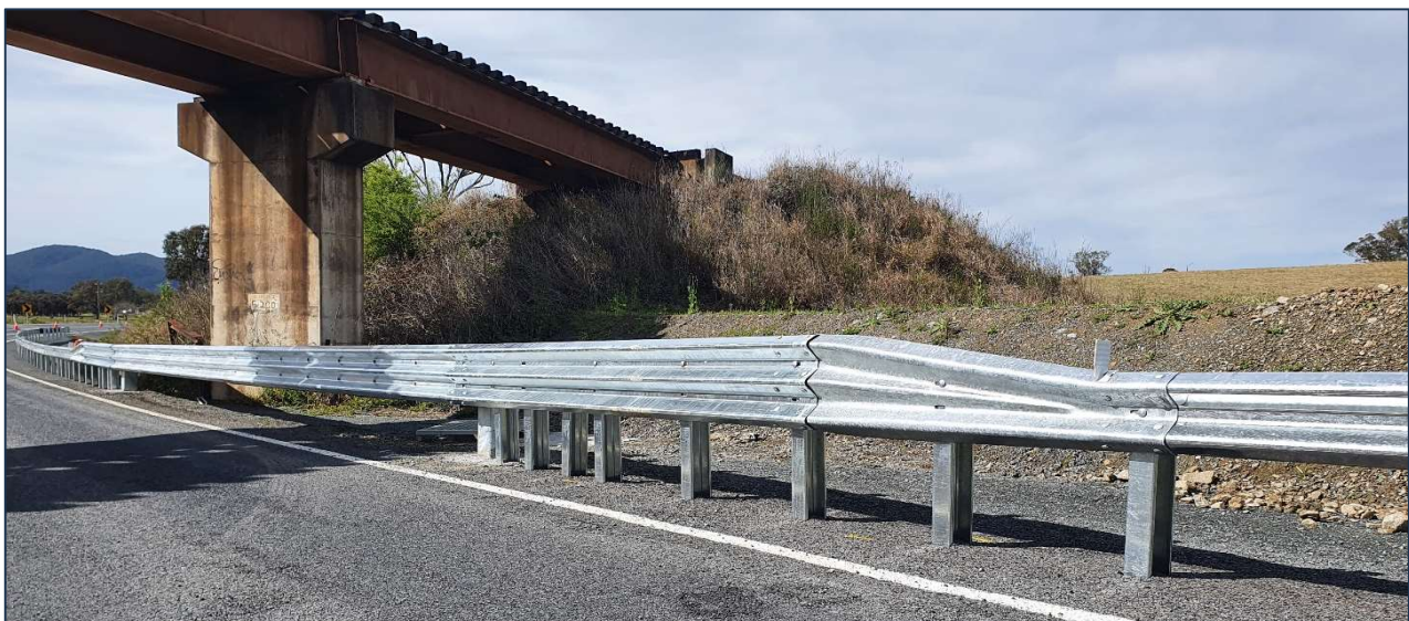
Figure 5: CrocGuard® Connection to RamShield® W-Beam
