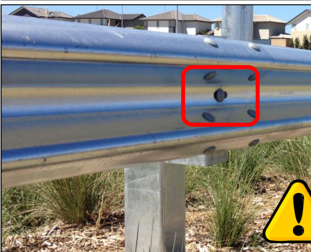
Figure 3: Design Limitations of G4 W-Beam with C-Blocks
