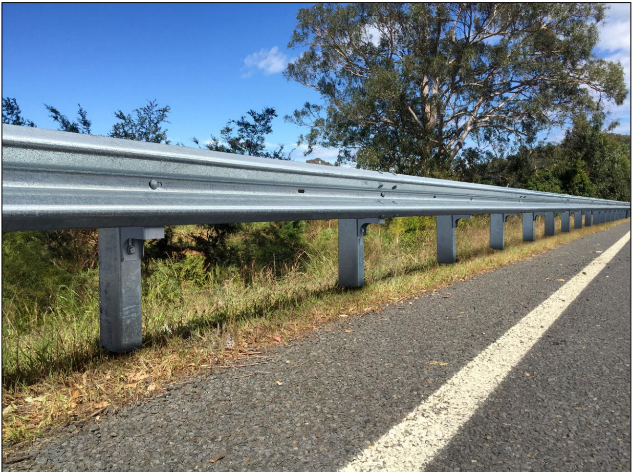
Figure 4: G4 W-Beam with RocketBloc™ - Front View
