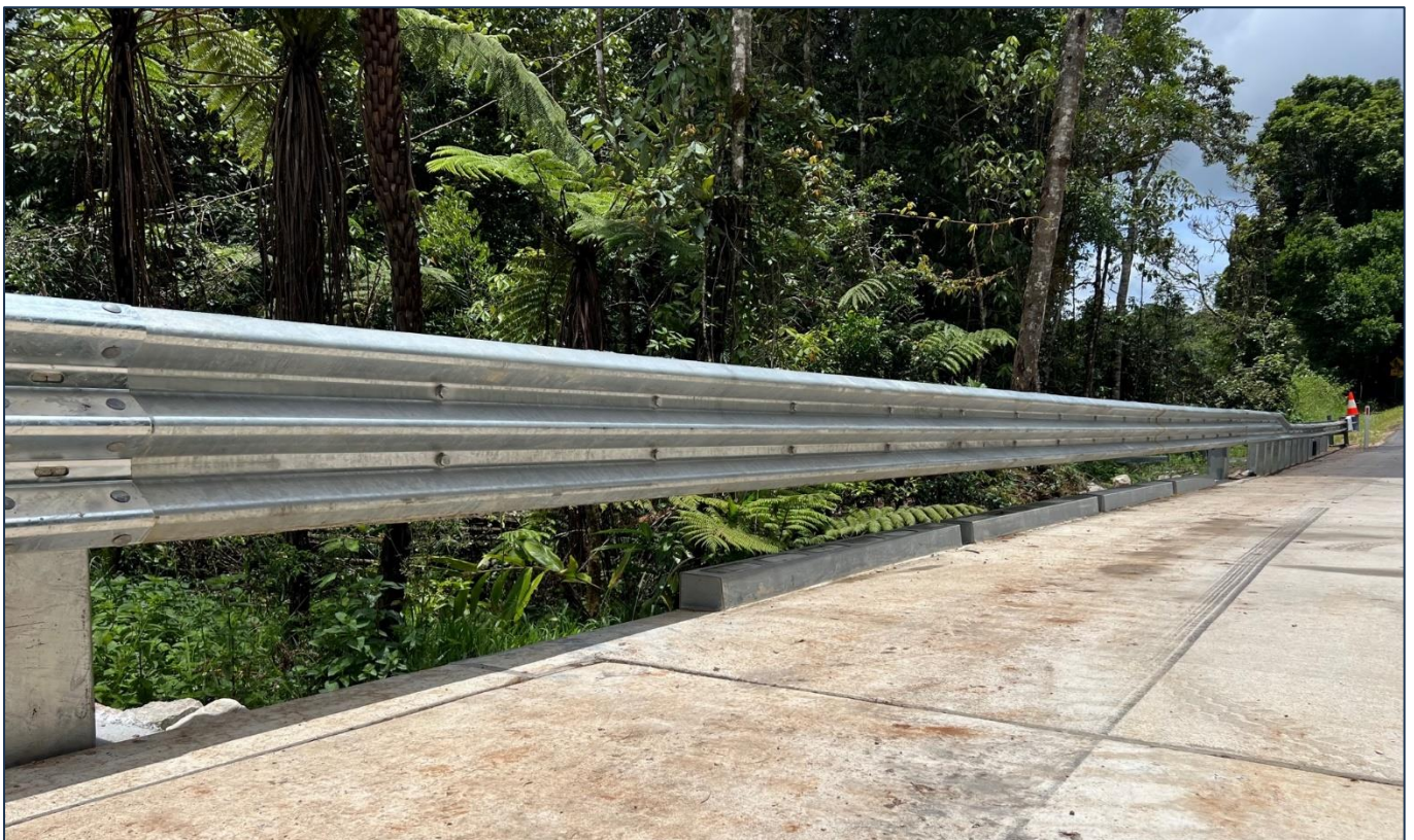
Figure 6: CrocGuard® Connection to RamShield® HC
