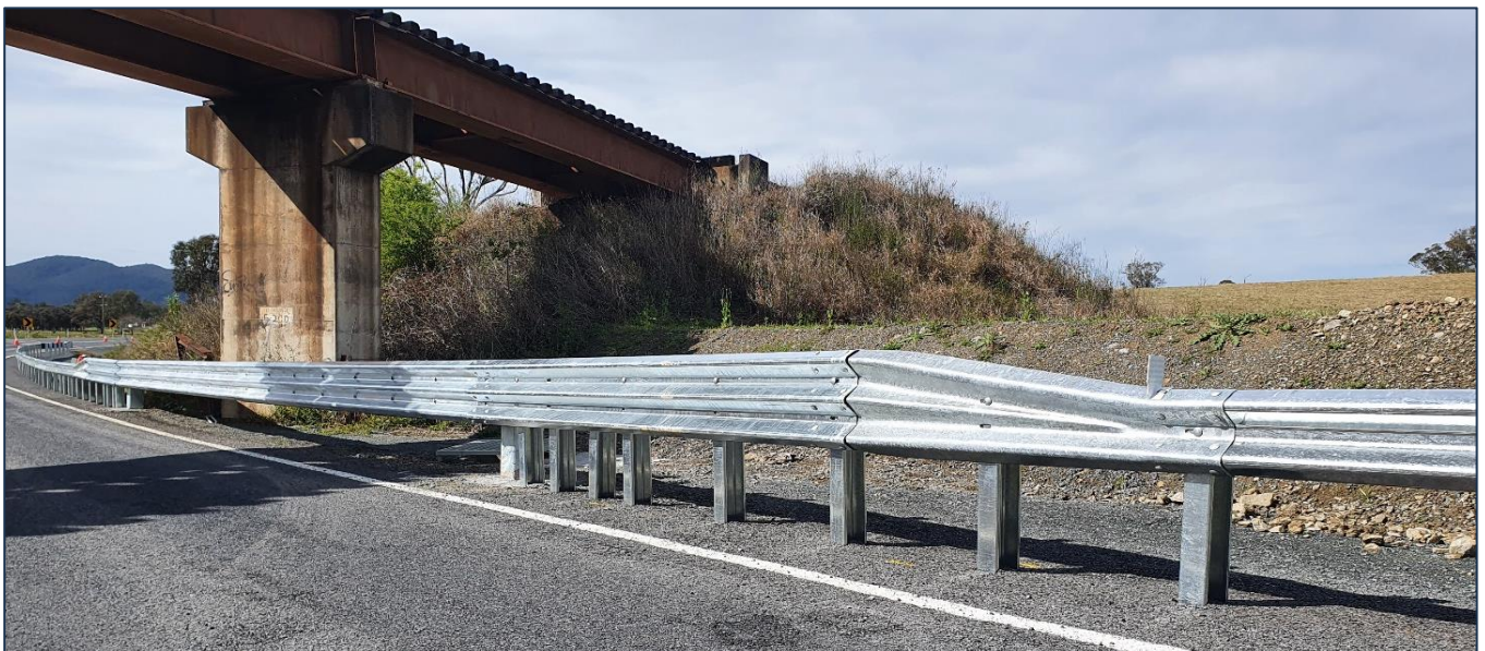
Figure 5: CrocGuard® Connection to RamShield® W-Beam
