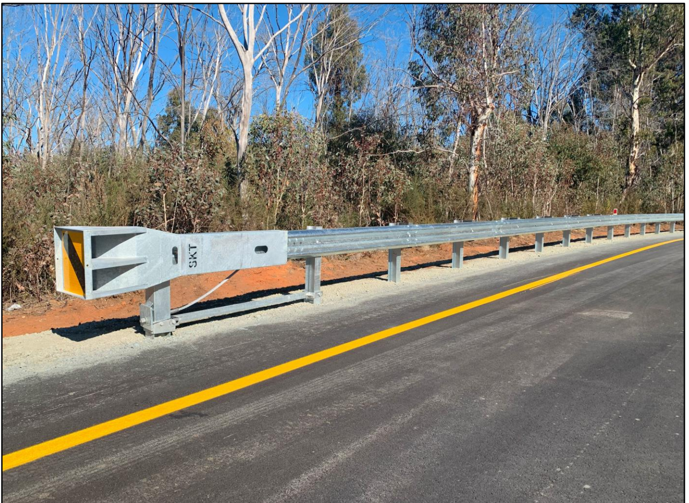
Figure 3: MSKT Terminal Connection to RamShield® Low Deflection
